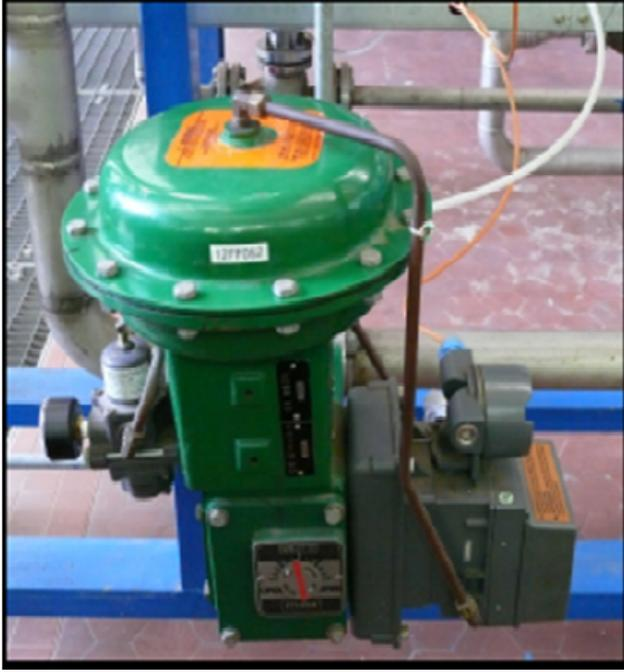
(a) Valve with pneumatic actuator.
