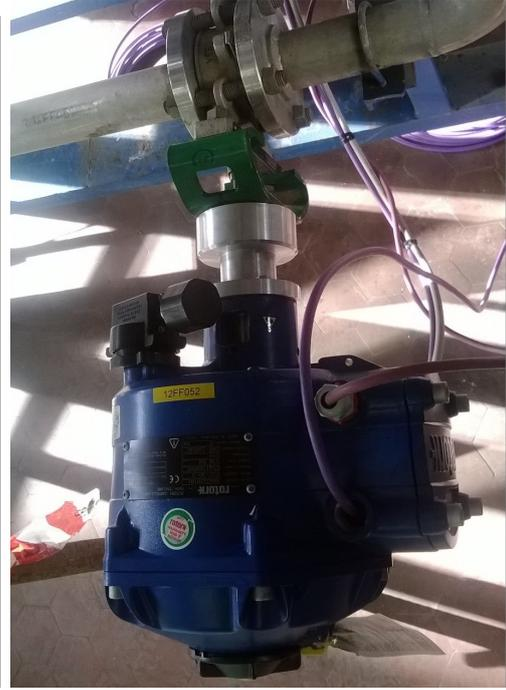
(b) Valve with electric actuator.
